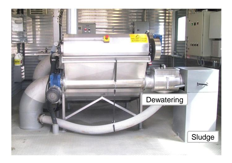
Reduced sludge volume from 2.8 to 0.2 gpm (0.2 to 0.01 L/s) Sludge DM increased from 1-2% to 20-25%
