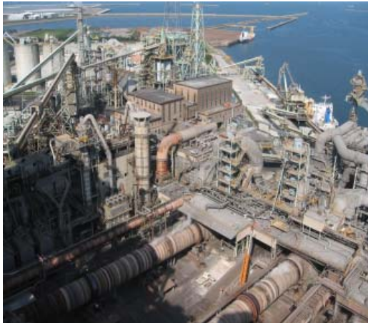
Mitsubishi Materials 15 types of waste treatment and recycling, such as metal waste and sludge
