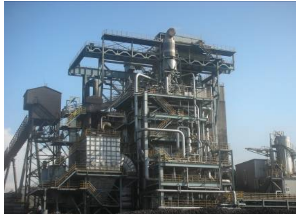
Nippon Coke & Engineering CDQ (Coke Dry Quenching Process) Supply power and steam to neighboring factories Power generation capacity: 27,900kW
