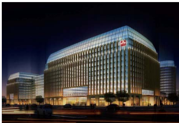
Huatai Securities Plaza Ground-source Heat Pump Central Air Conditioning System
