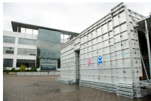
PreMold Aluminum Formwork
