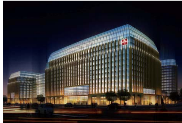
Huatai Securities Plaza Ground-source Heat Pump Central Air Conditioning System
