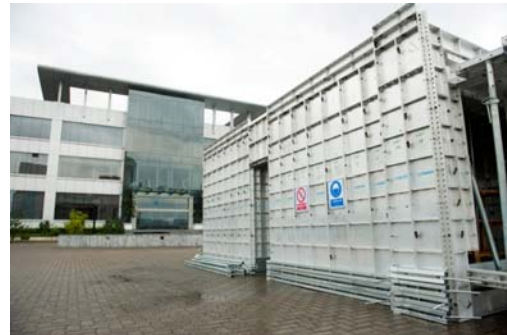
PreMold Aluminum Formwork
