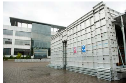
PreMold Aluminum Formwork
